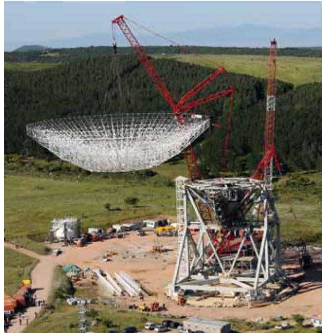
Assembly work on the radio telescope in Sardinia
